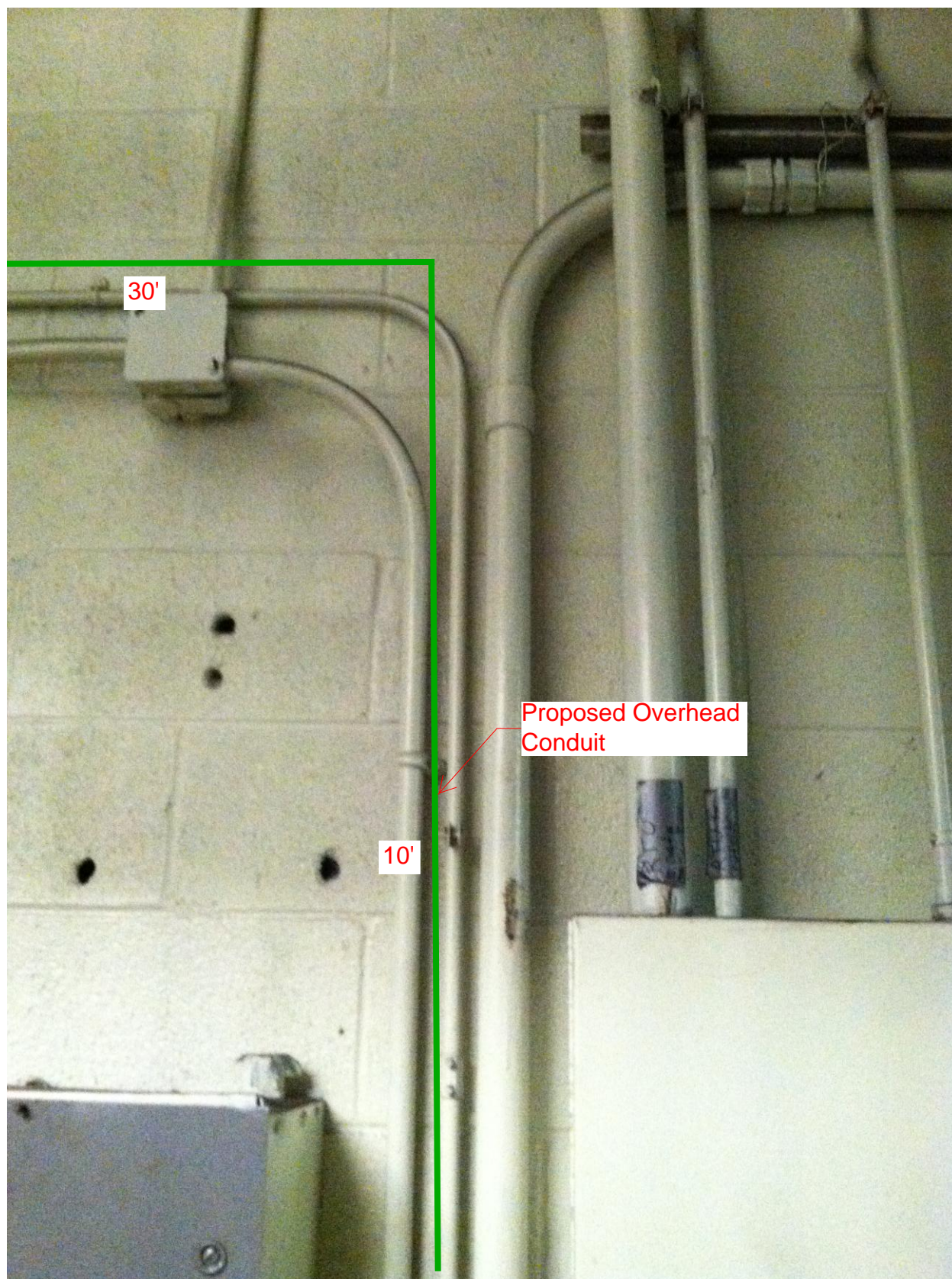
Photo #8: Proposed Overhead Conduit in Room W202.
