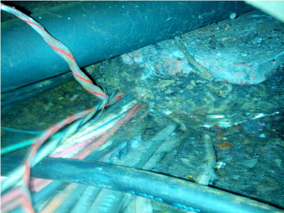
Photo #4: B06 Fort Totten – Pull string installed in power duct run from handhole to kiosk
