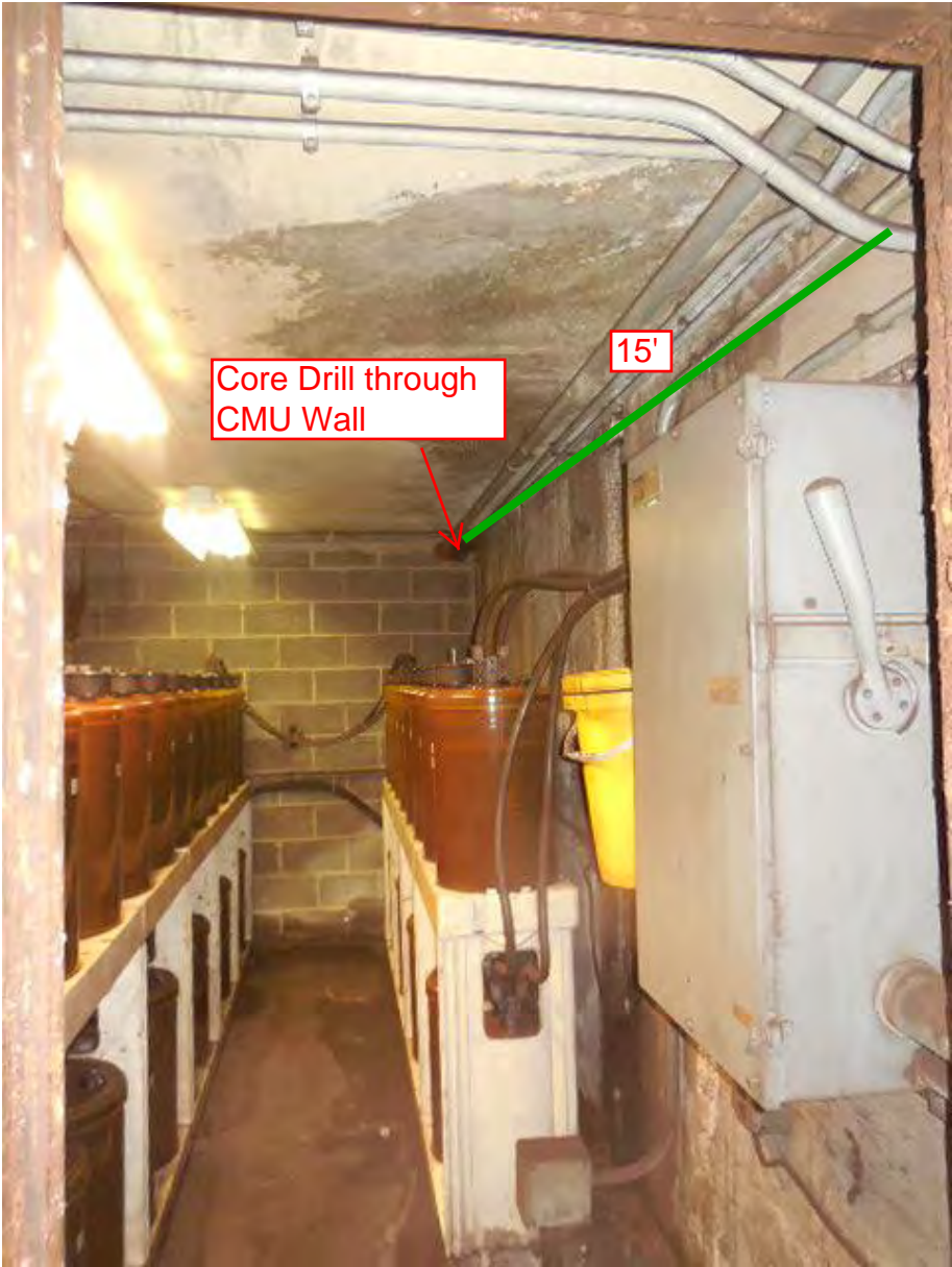
Photo #8 – Proposed Overhead Conduit in Battery Room 218
