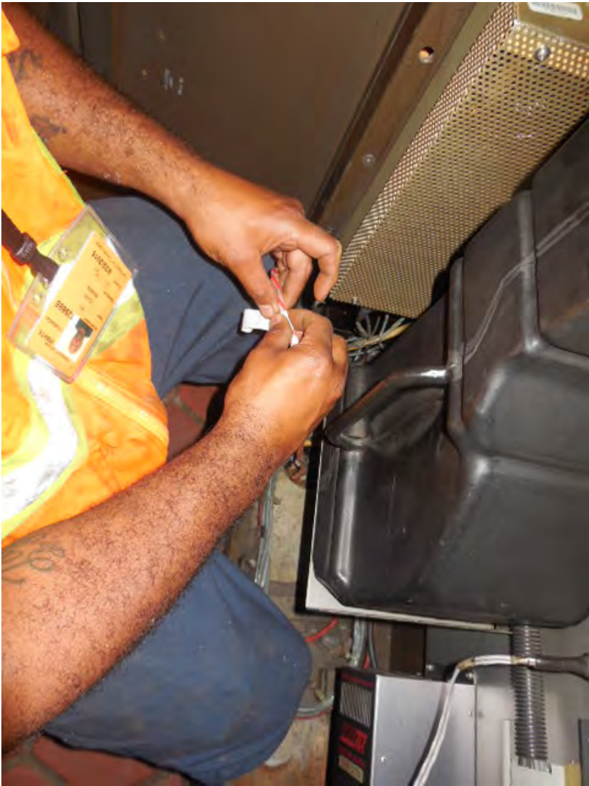
Photo #9: A13 Twinbrook – Installation of pull string in faregate array ducts
