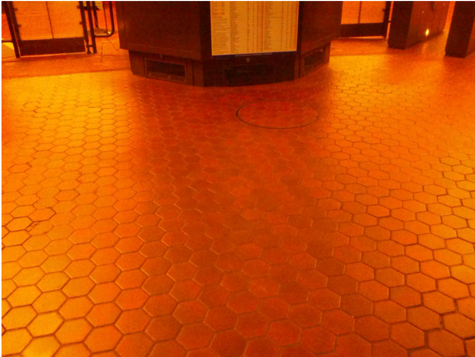
Photo #1: Kiosk on mezzanine floor
