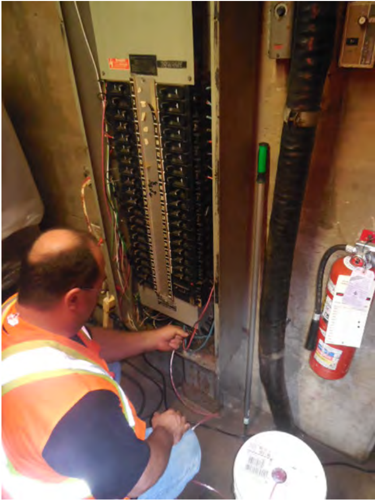
Photo #6: A12 White Flint – Pull string installation in AFC panel from kiosk
