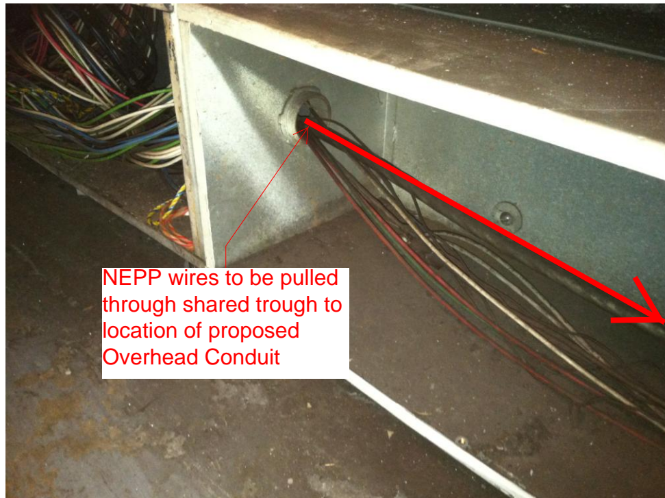
Photo #6: NEPP wires to be pulled through Shared Trough in Room W202.
