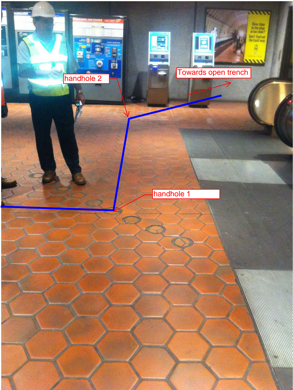
Photo #2 – A05 Cleveland Park: Handhole 1 and Handhole 2
