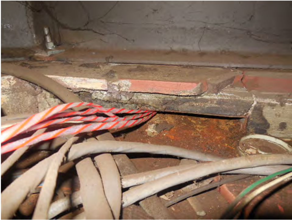
Photo #2: A12 White Flint – Pull string installation in faregate array duct
