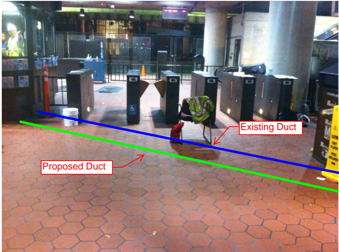
Photo #2 – Proposed and existing ducts on mezzanine floor
