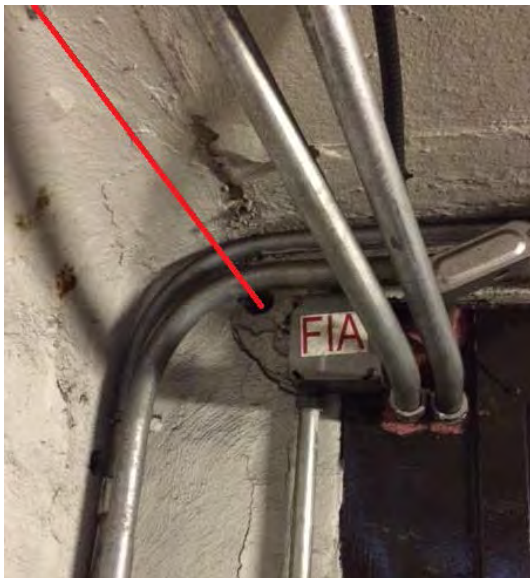
Farragut North NW Photo # 9 – Proposed conduit run through existing core drill
