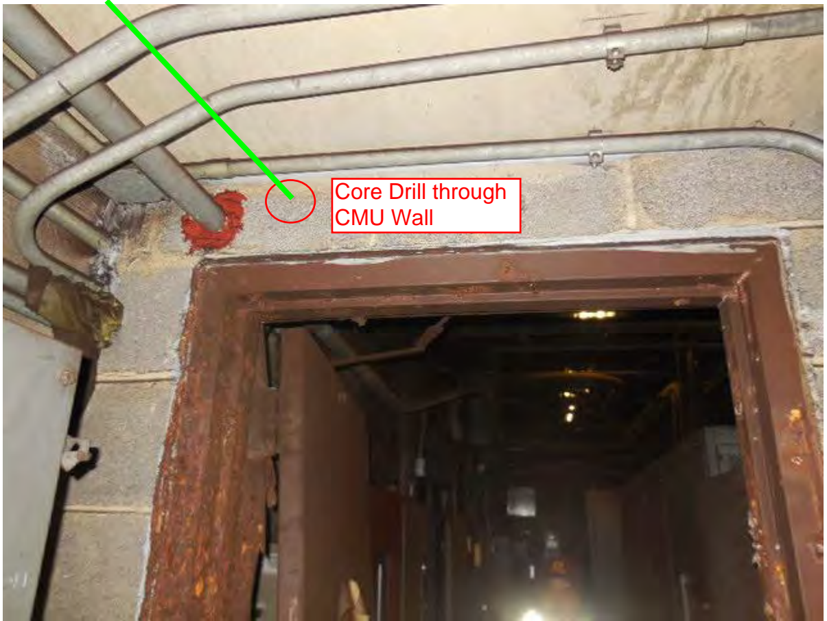
Photo #9 – Proposed Overhead Conduit in Battery Room 218
