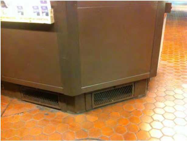
Farragut North NW Photo # 4 – Kiosk floor, there is a skirt obstruction inside Kiosk and a narrow gap for wires
