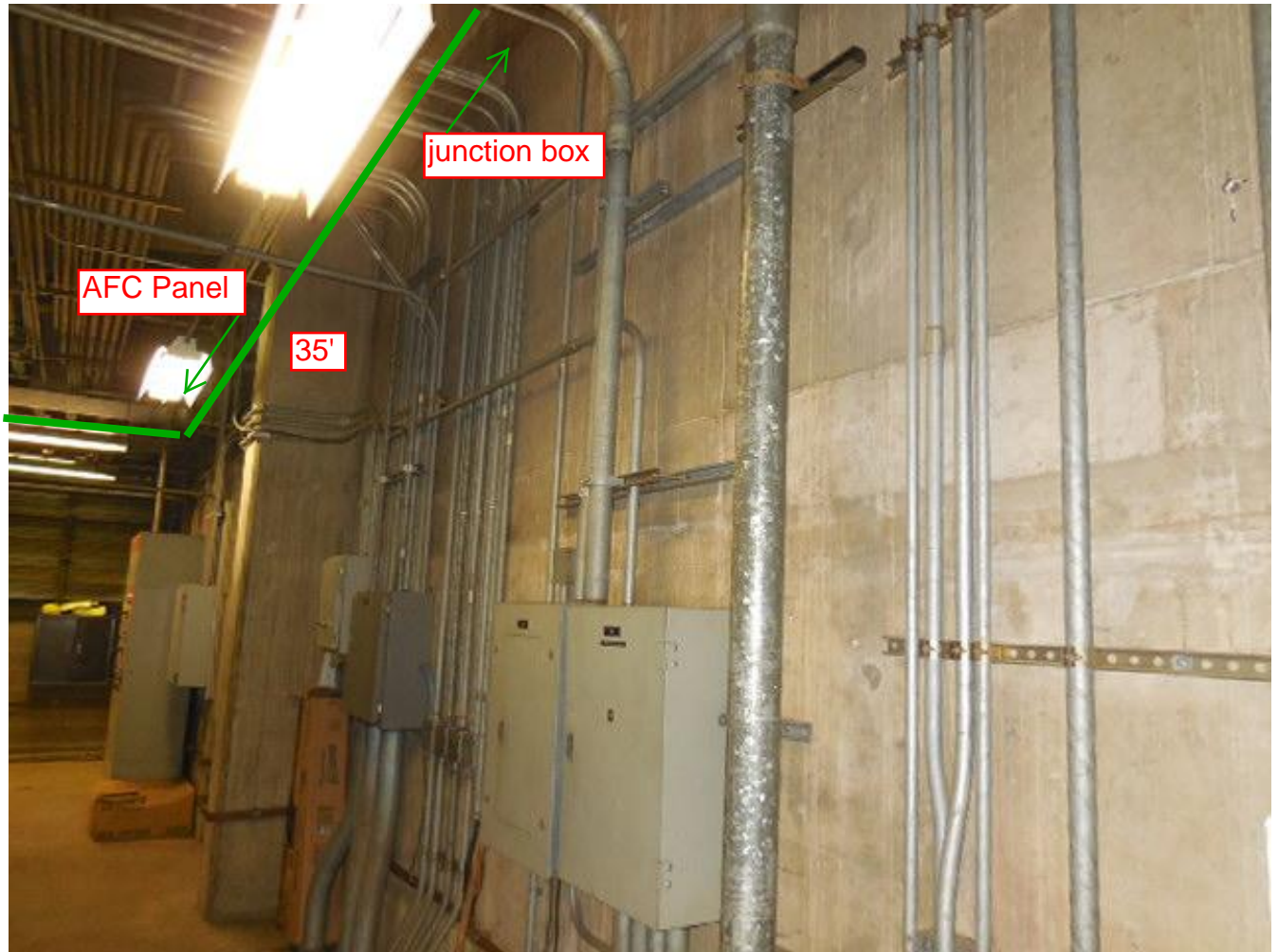
Photo #9 - Proposed conduit run inside Room C106
