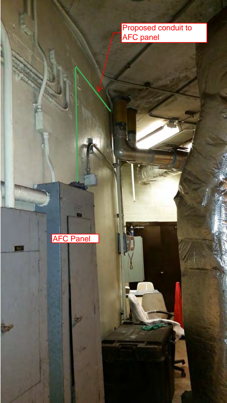
Photo #6: Proposed conduit run to AFC panel
