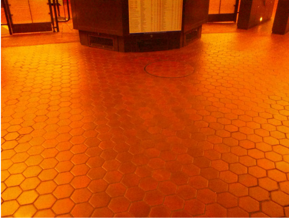
Photo #1: Kiosk on mezzanine floor
