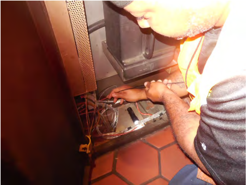
Photo #8: A13 Twinbrook – Inserting fish tape into faregate array ducts
