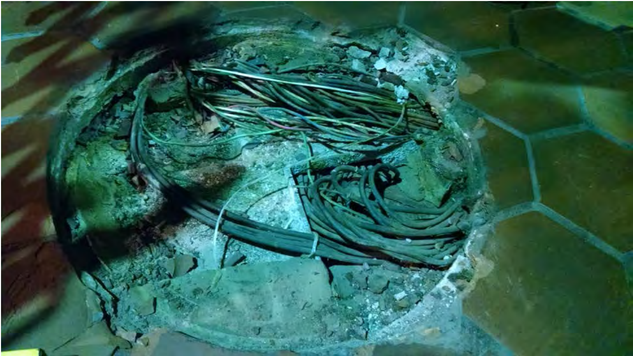
Photo #4: B06 Fort Totten – Pull string installed in power duct run from handhole to kiosk
