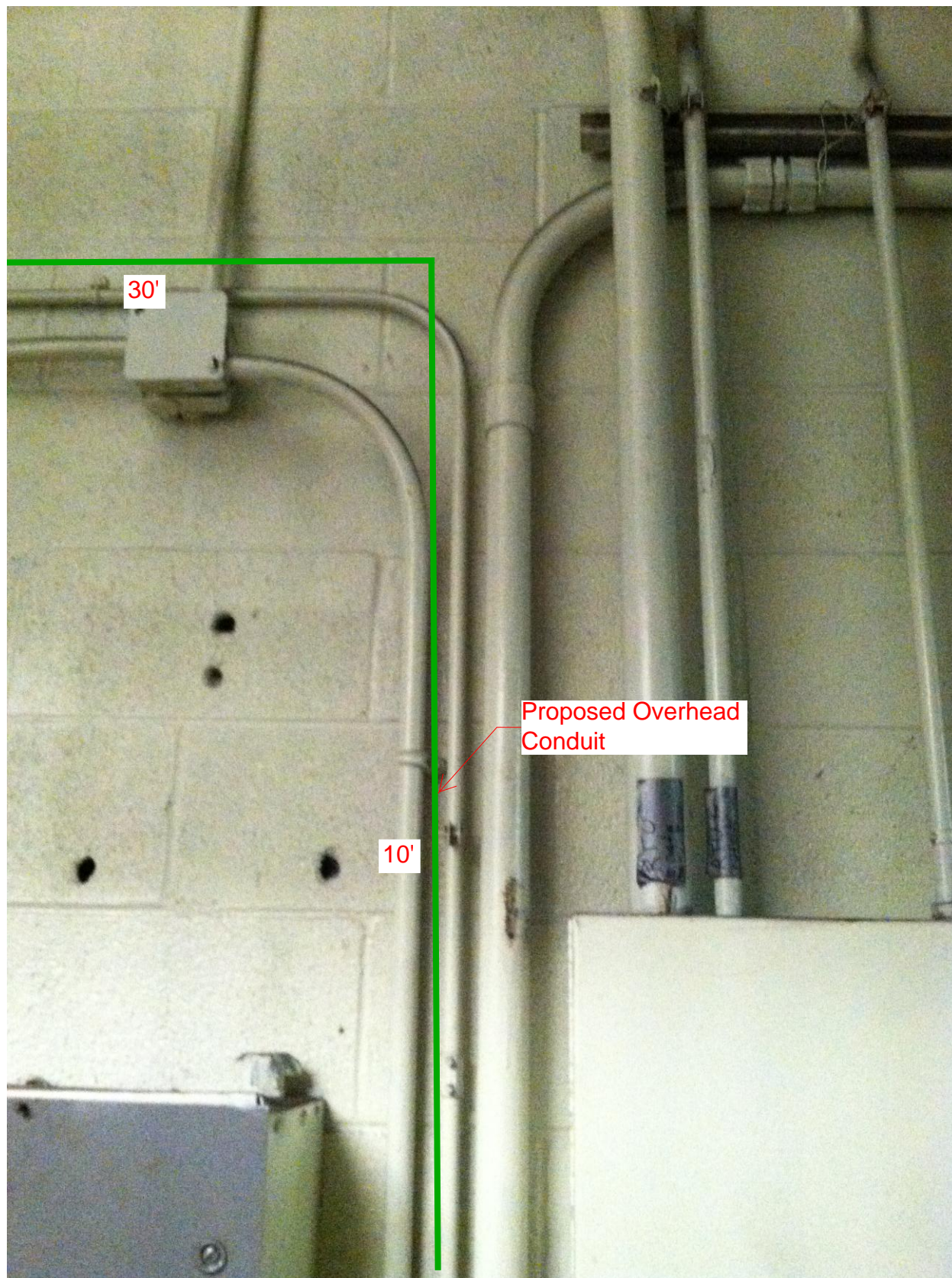
Photo #8: Proposed Overhead Conduit in Room W202.
