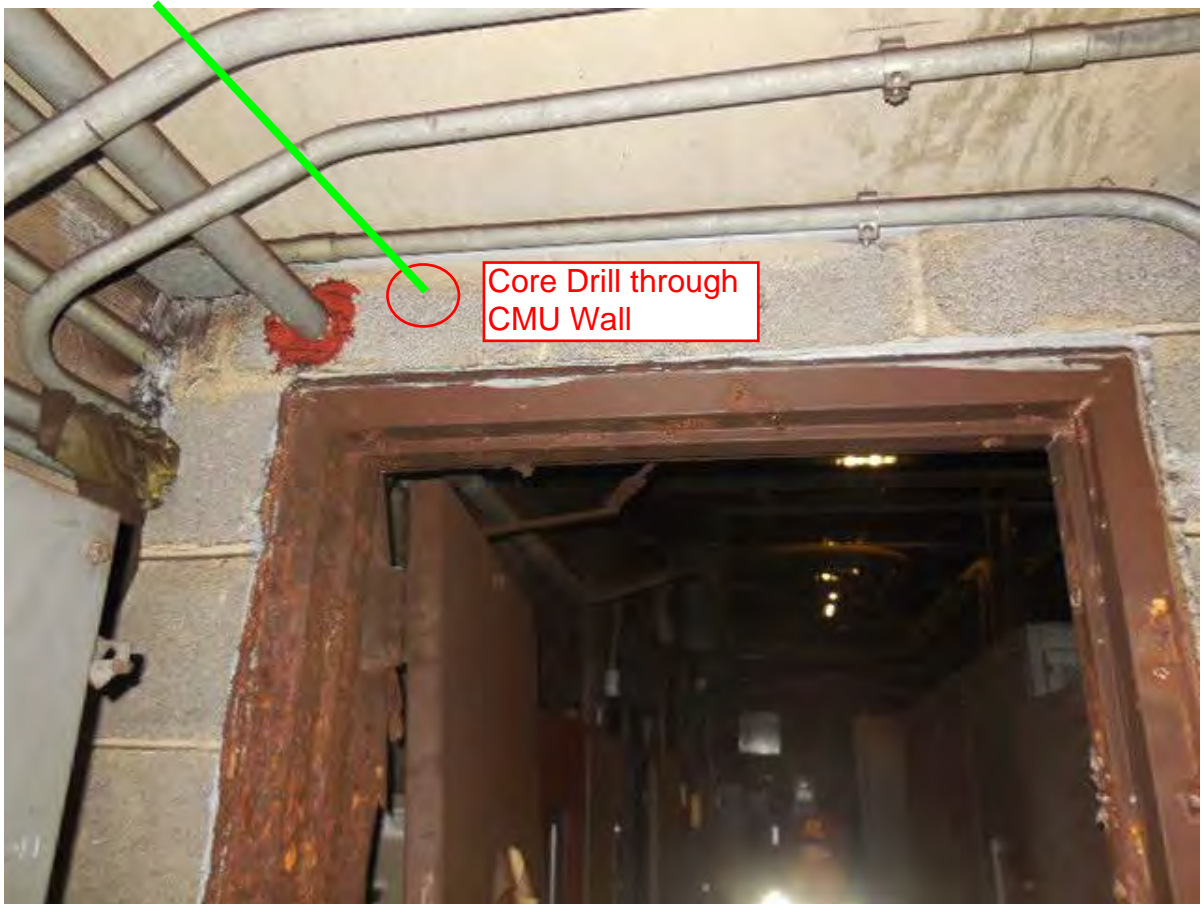
Photo #9 – Proposed Overhead Conduit in Battery Room 218
