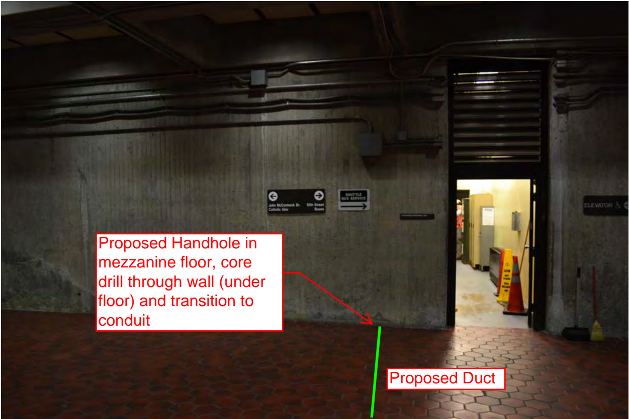
Photo # 5 – Proposed duct approach to back rooms
