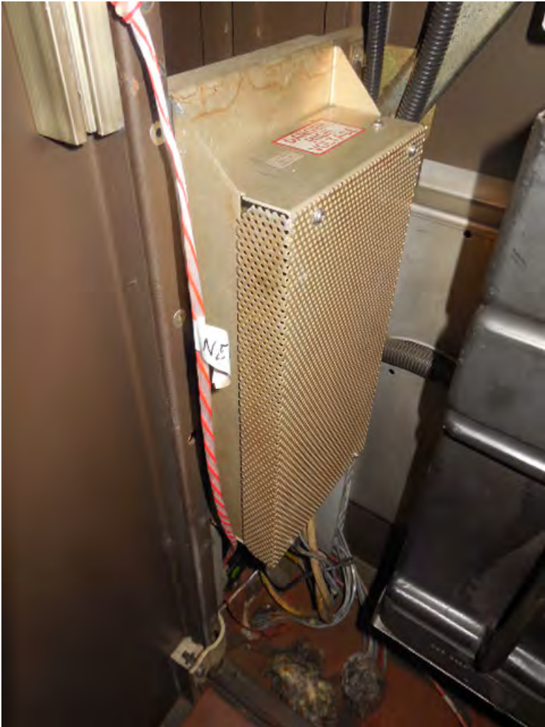
Photo #4: A12 White Flint – Pull string installation in faregate
