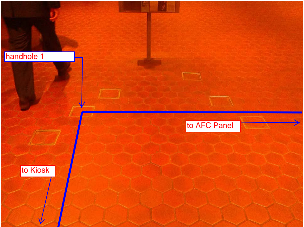
Photo #1 – A01 Metro Center West: Mezzanine level handholes
