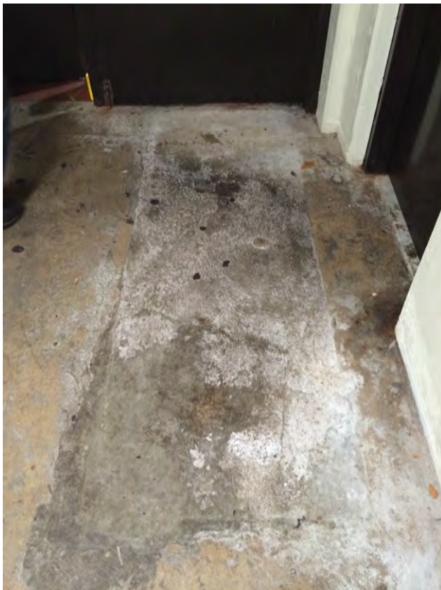
Rockville Photo #3 – Concrete repair to floor in back hallway outside Room C113
