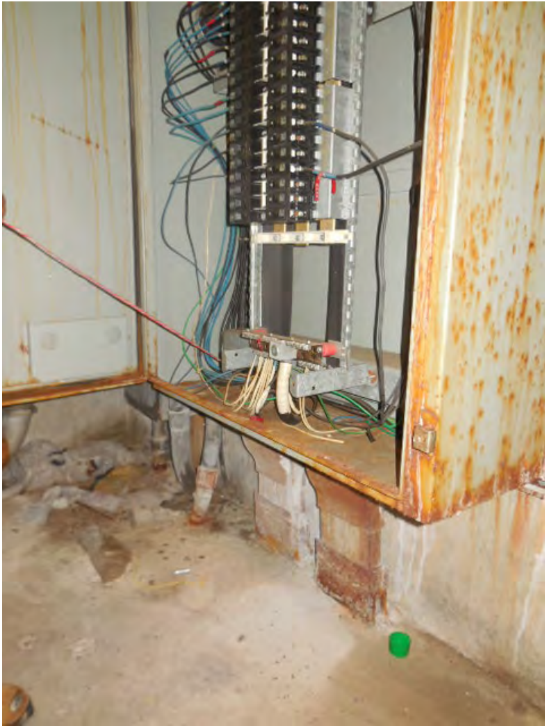
Photo #3: A13 Twinbrook – Pull string installation to AFC Panel
