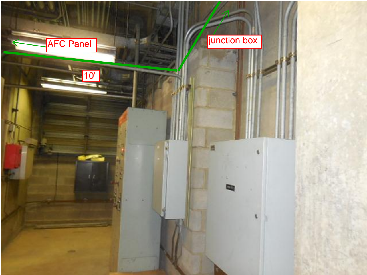
Photo #10 - Proposed conduit run inside Room C106
