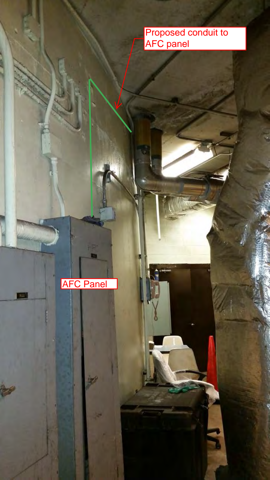
Photo #6: Proposed conduit run to AFC panel
