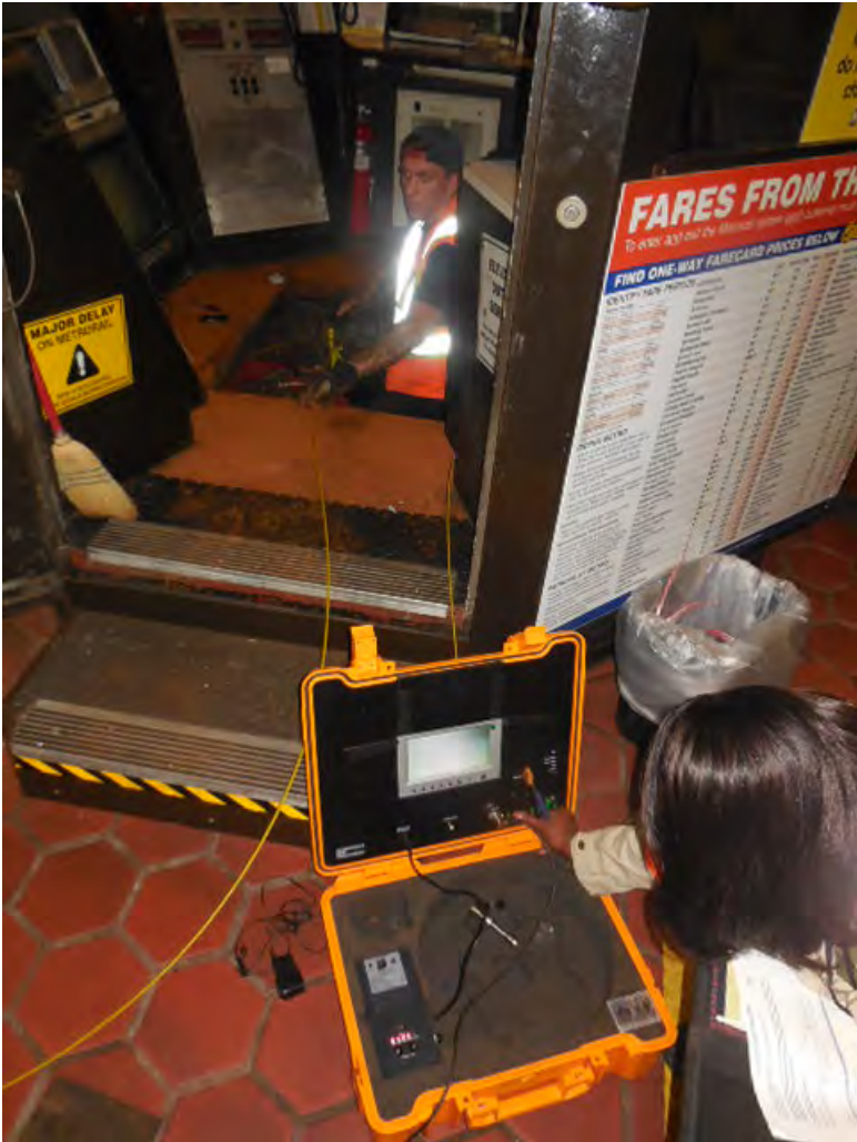
Photo #5: A12 White Flint – Video-scoping faregate array ducts
