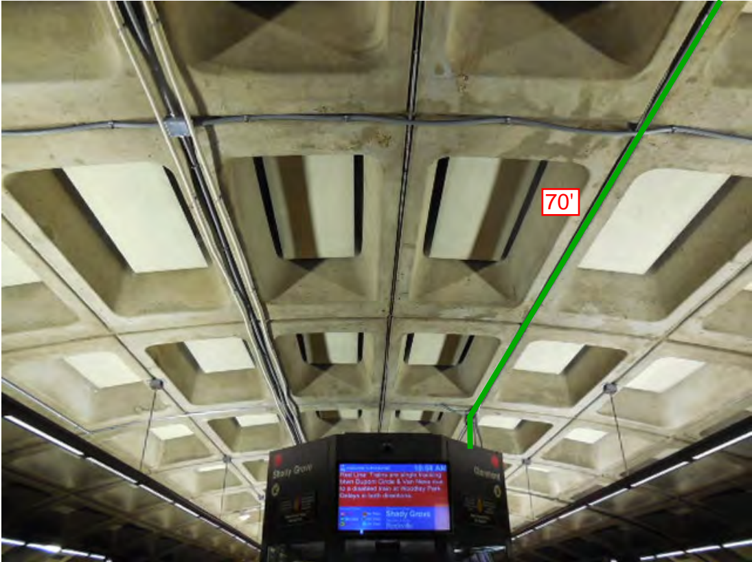
Photo # 4 – Proposed Conduit Run
