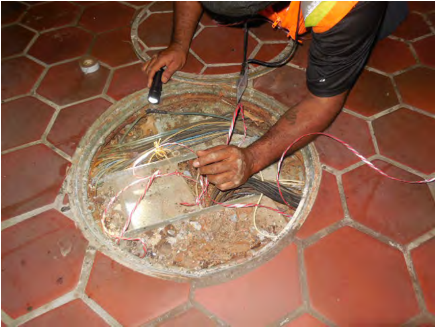
Photo #5: A13 Twinbrook – Pull string installation to mezzanine handhole
