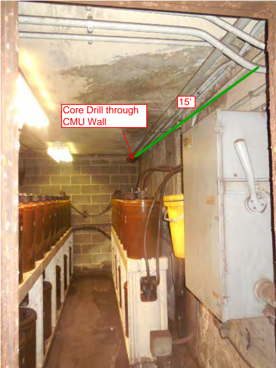
Photo #8 – Proposed Overhead Conduit in Battery Room 218
