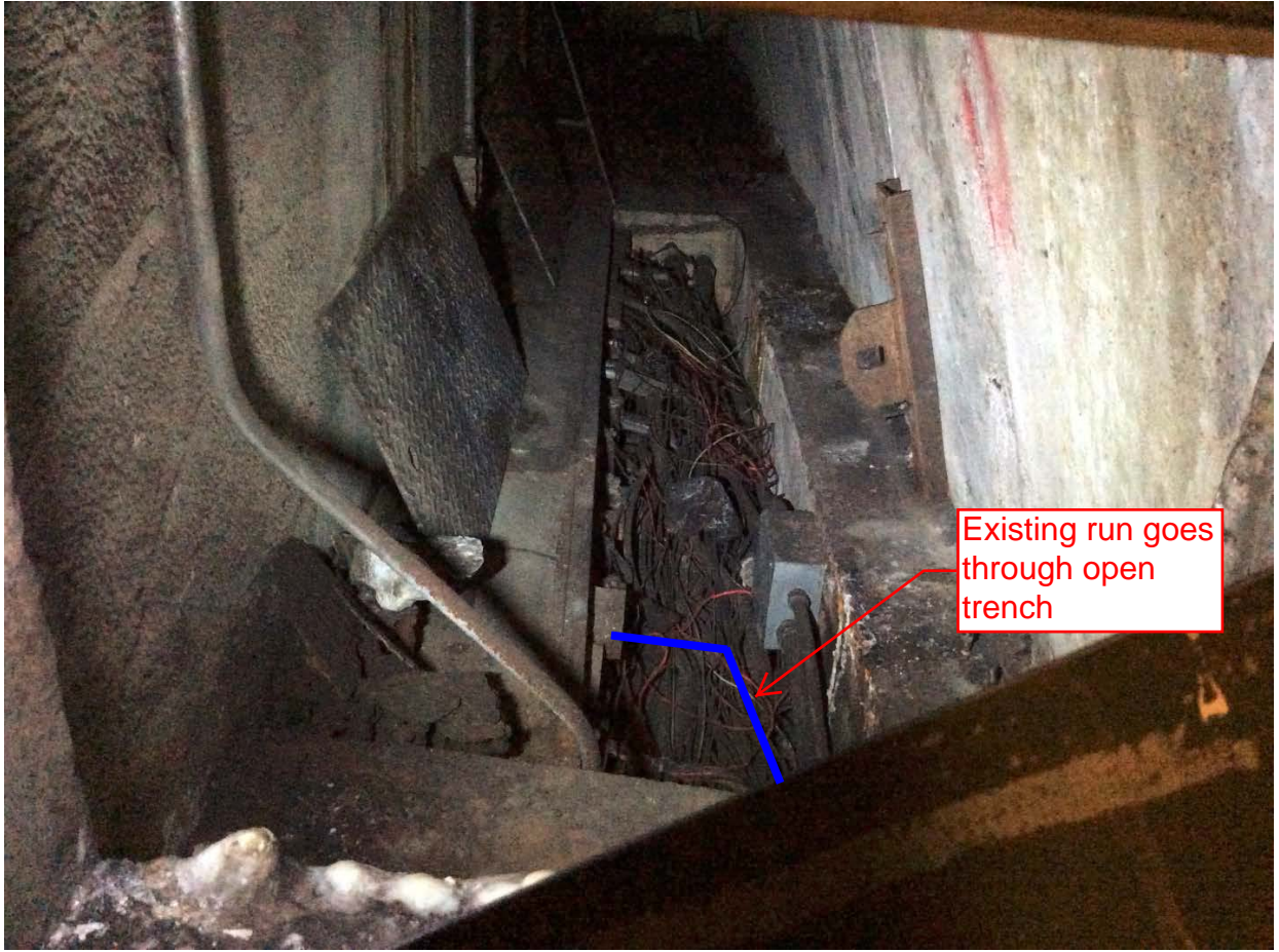
Photo #3 – A05 Cleveland Park: Existing power run in open trench
