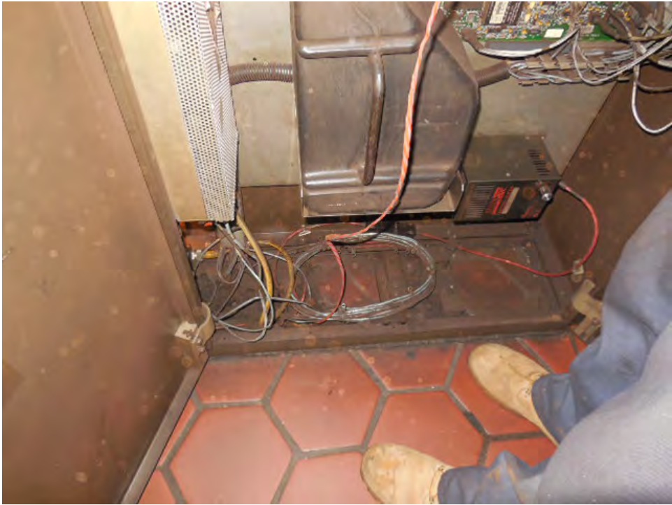
Photo #3: A08 Friendship Heights – Pull string installed in faregate array duct
