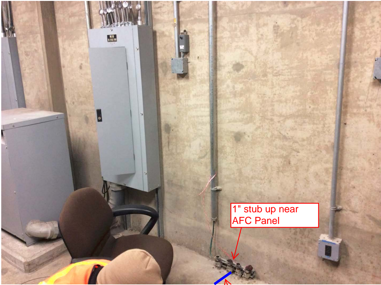
Photo #3 – B35 New York Ave South: AFC Panel near 1 inch stub up
